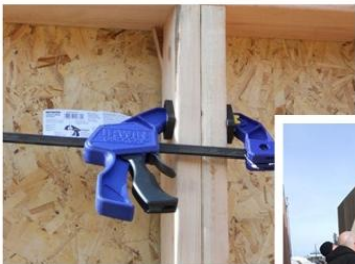
Be sure it laps over the corner panel's seams.
